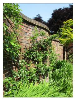
The wavy wall at the bottom of the kitchen garden is a charming feature which blends aesthetics and practicality. The undulations may have been designed to provide shelter for tender plants, but they also lend stability to the wall, avoiding the need for buttresses.
